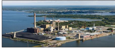
Central Energy Plant
